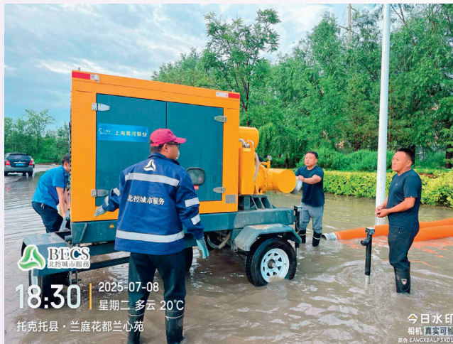
Flood Relief Site
