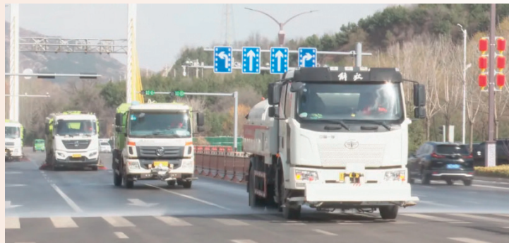
Water Sprinkling and Dust Suppression Operations at the Heshun Project
